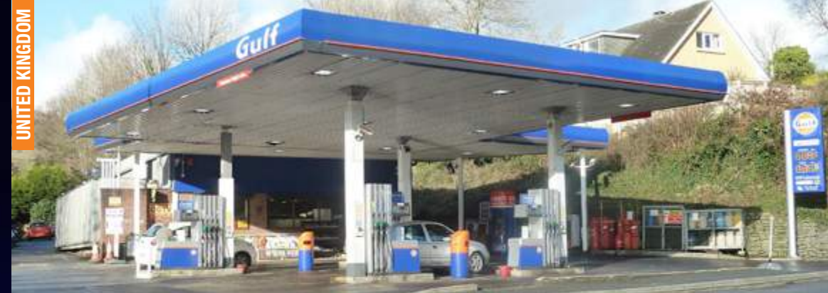
The six million litres per annum Tanderdy Garage, Carmarthen, one of 18 new additions to the Gulf network in the UK
